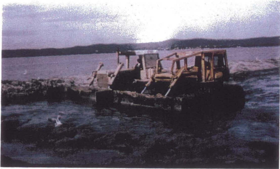
Figure 62. Swamp dozers removing sediment and macrophytes as part of the restoration project
