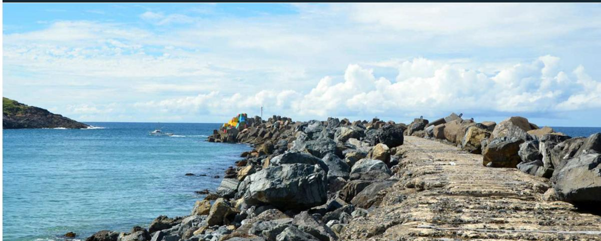
Across the eastern seaboard of Australia, breakwaters and training walls have instigated fundamental perturbations to coastal and estuary processes. This has induced long-term changes to foreshore alignments, tidal currents, tidal planes and marine ecologies, with significant consequences. These effects can be seen right along the NSW coast of Australia, where breakwaters and training walls have been implemented.
