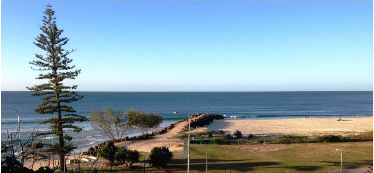
Kirra Point Groyne, Qld (Photo 07/07/2013,
