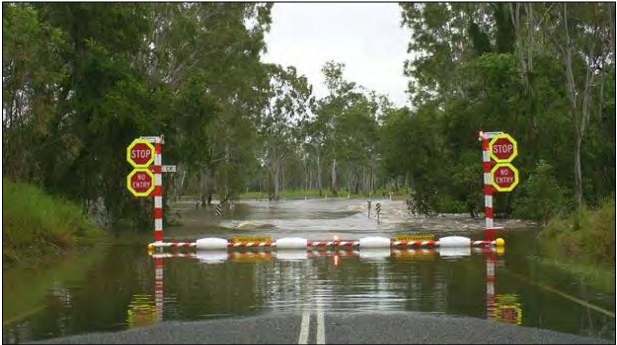
Plate 19 Examples of automatic flood gate system (photo courtesy of David Bagnall)
