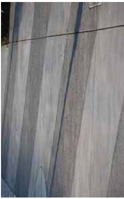
Shot blast concrete footpath
